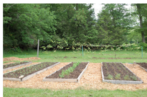
Newly constructed raised beds with culinary herbs.
